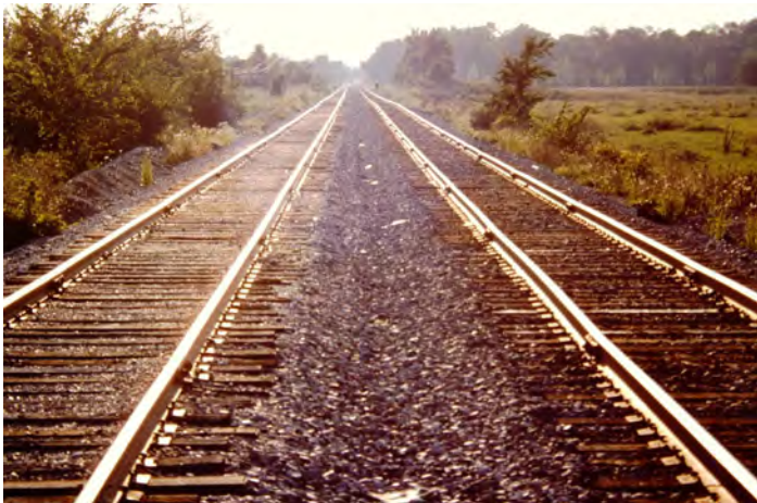
Mainline track, showing slope of ballast and drainage between tracks.
