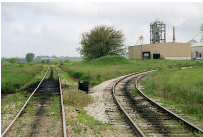
Oil soaks the ties and ballast where a locomotive is generally parked on the Iowa River Railway near Steamboat Rock, IA.
