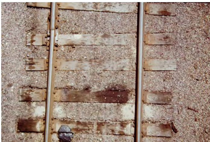
Chips of pink lady ballast in Butler Yard, with ballast to the tops of the ties for easy walking by trainmen.
